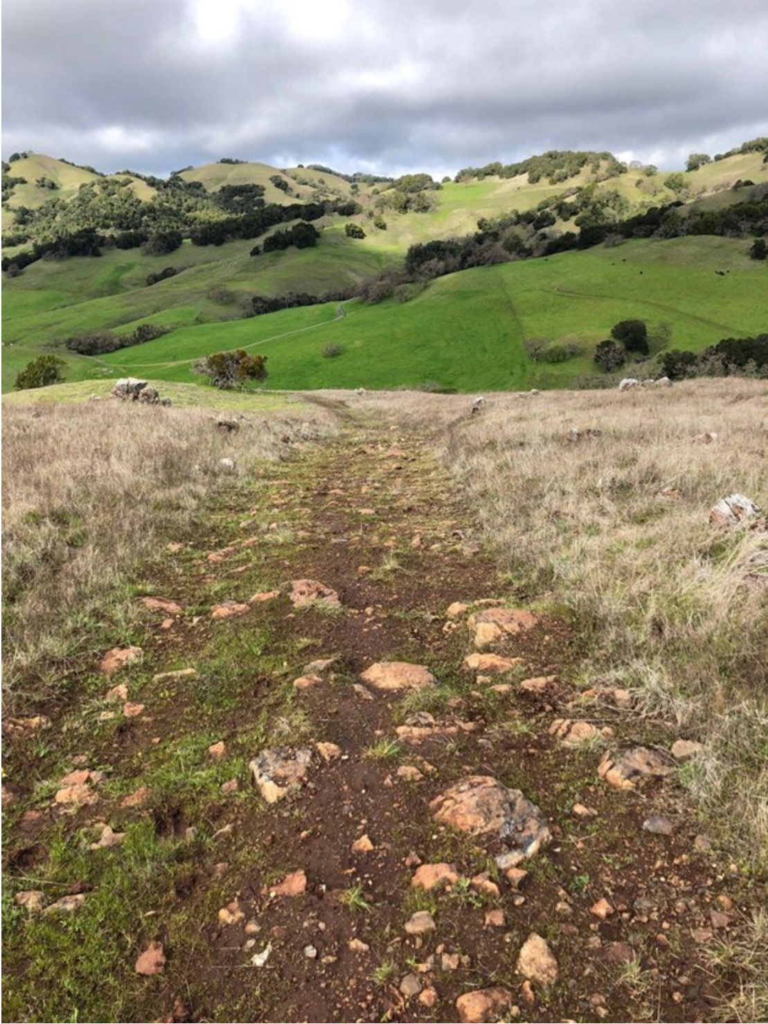
Photo 2. Fall-line through-cut segment of Upper Serpentine Road
