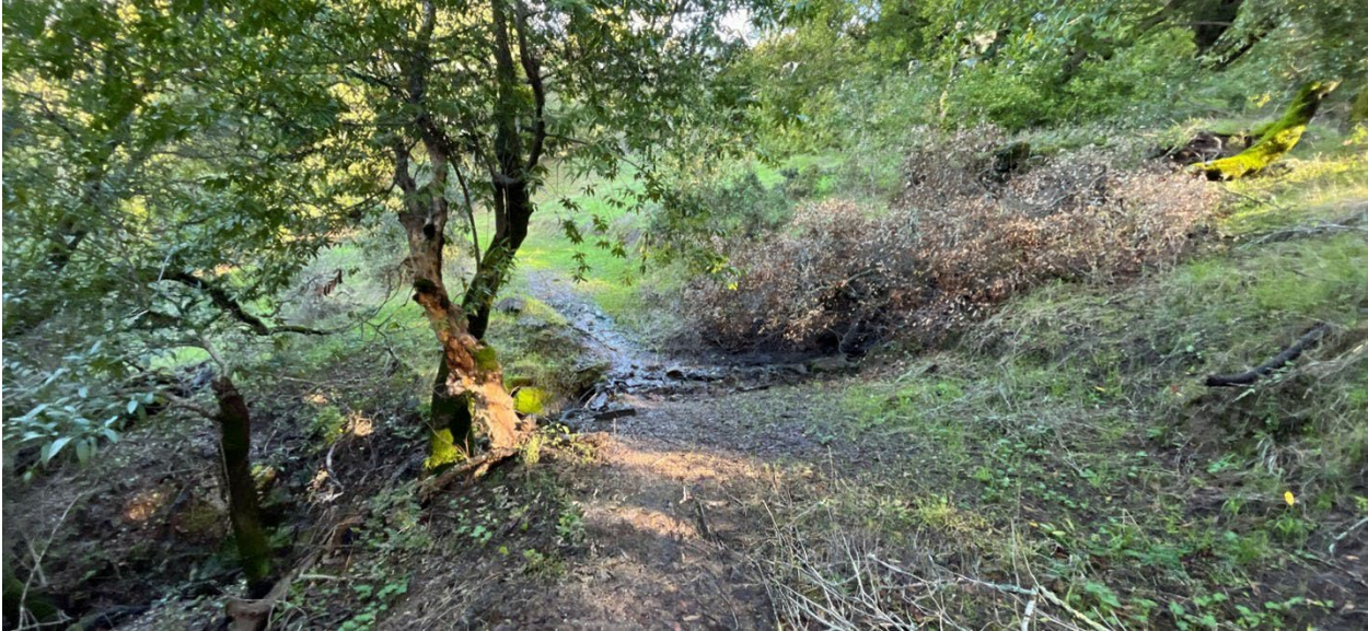
Photo 15. Road WB-05 at WC-16, proposed for removal and restoration
