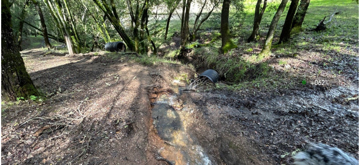
Photo 13. WC-15, proposed for removal and restoration
