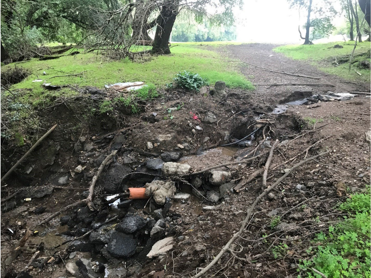
Photo 5. Watercourse crossing 5 (WC-05)
