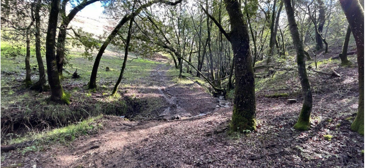
Photo 9. WC-10, proposed for removal and restoration
