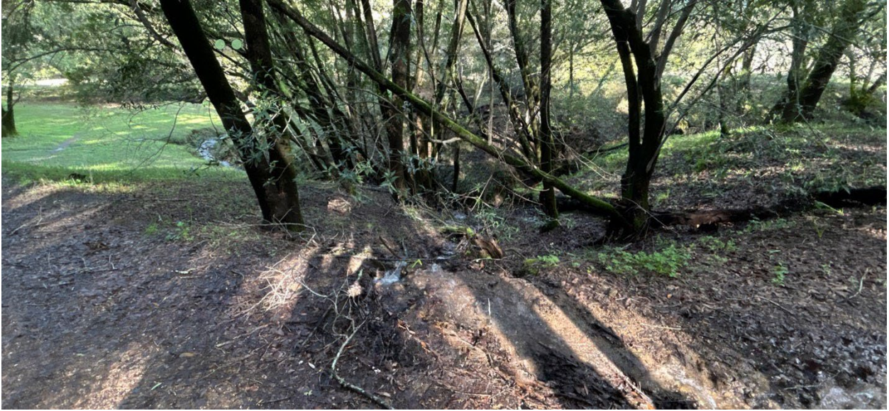
Photo 12. WC-13, proposed for removal and restoration
