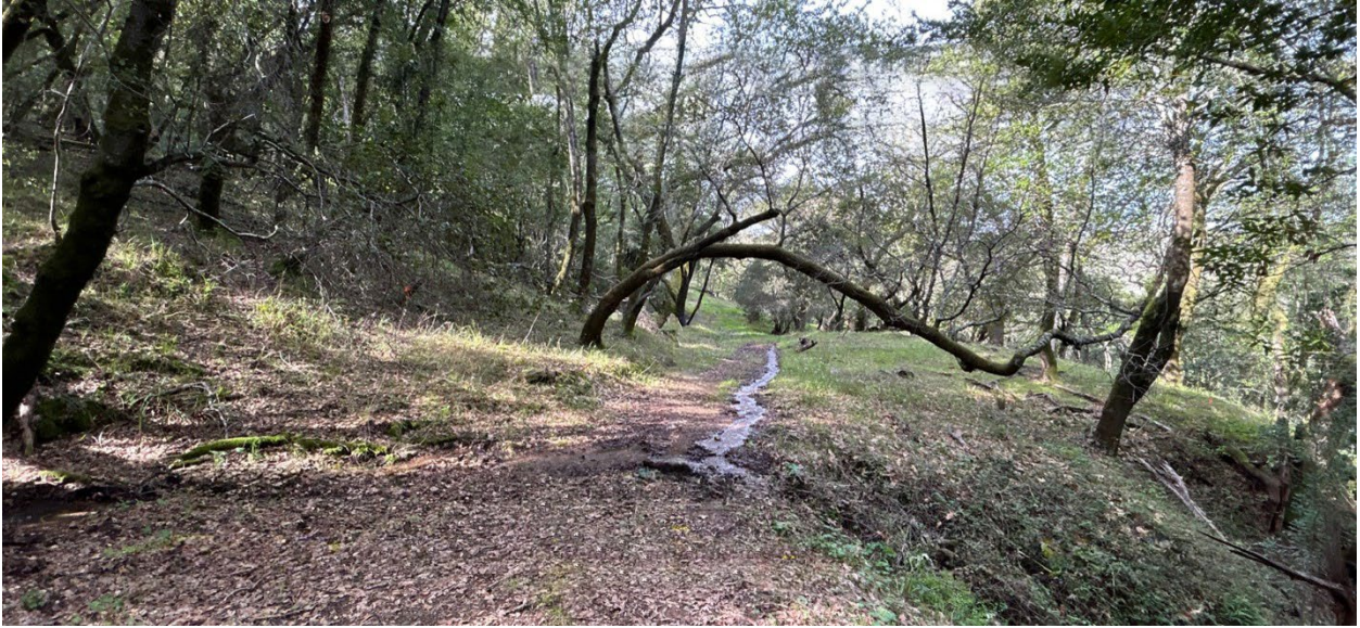
Photo 4. Road WB-02 at WC-8, showing stream flows currently diverted down the road.
