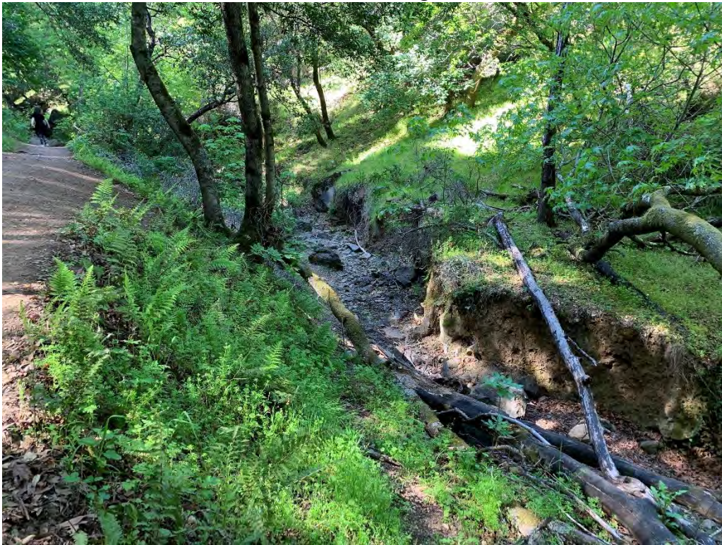
Incised channel along existing trail
