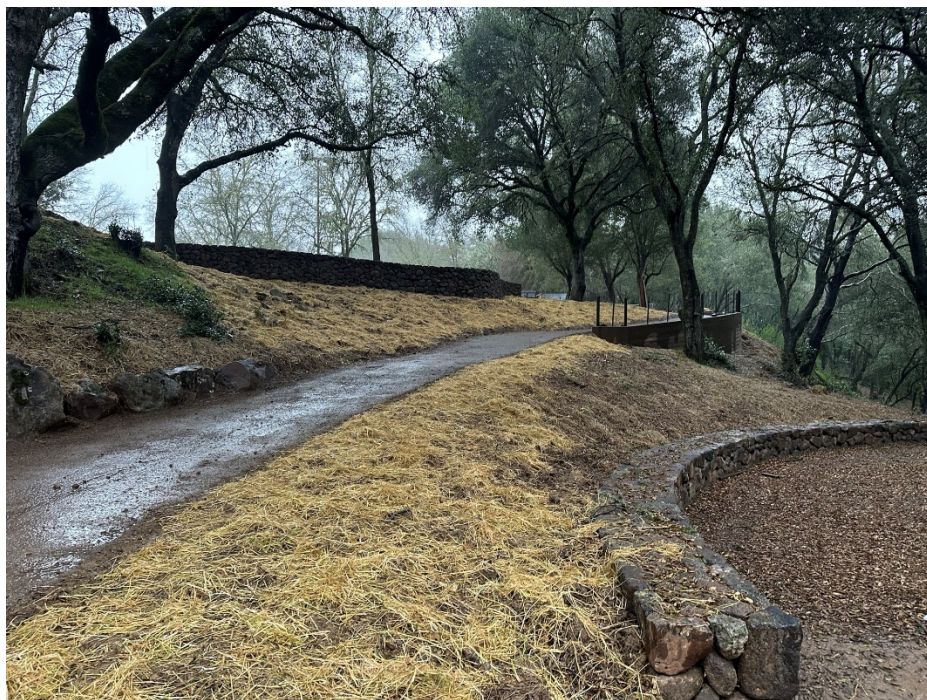
Photo 2. Example of a switchback trail in construction from Fitch Mountain
